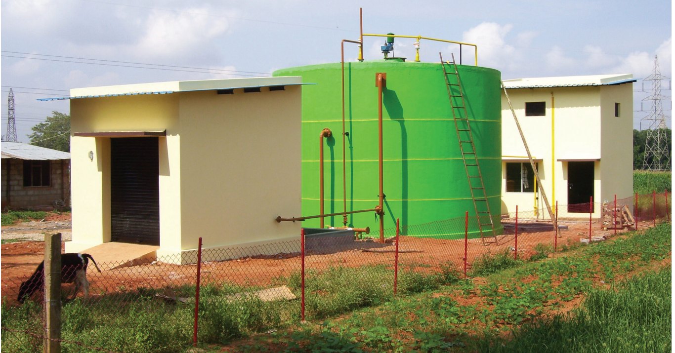
Mailhem's biogas plants for heat generation
